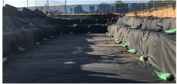
Field example of protected liner installation prior to module placement
